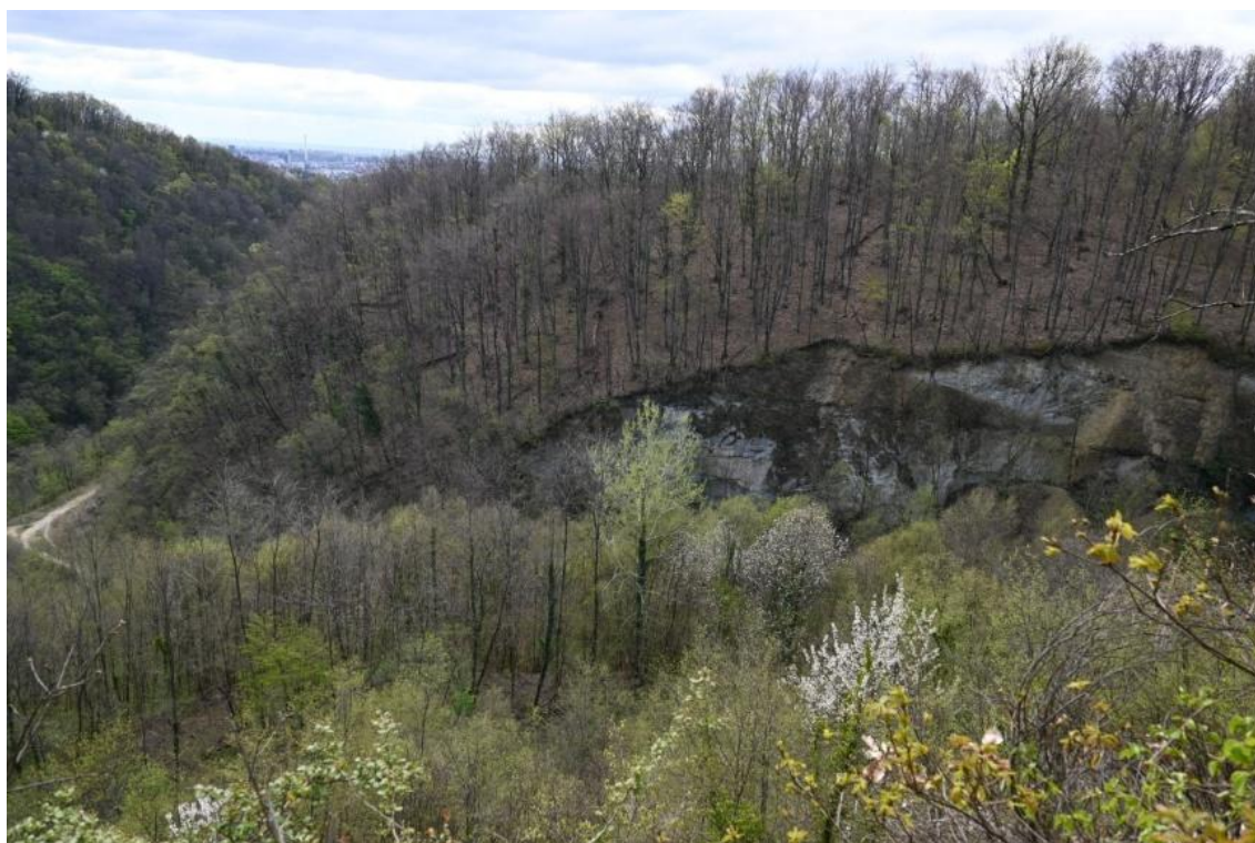
Figure 4. The current appearance of the Vrapče quarry, from which most of the stone material came during Bolle's renovation.
