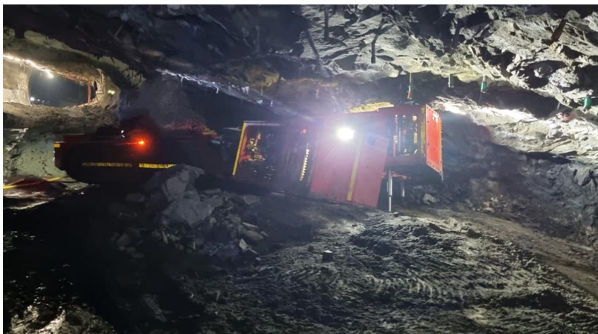
Figure 4. NRE support rig in operation
