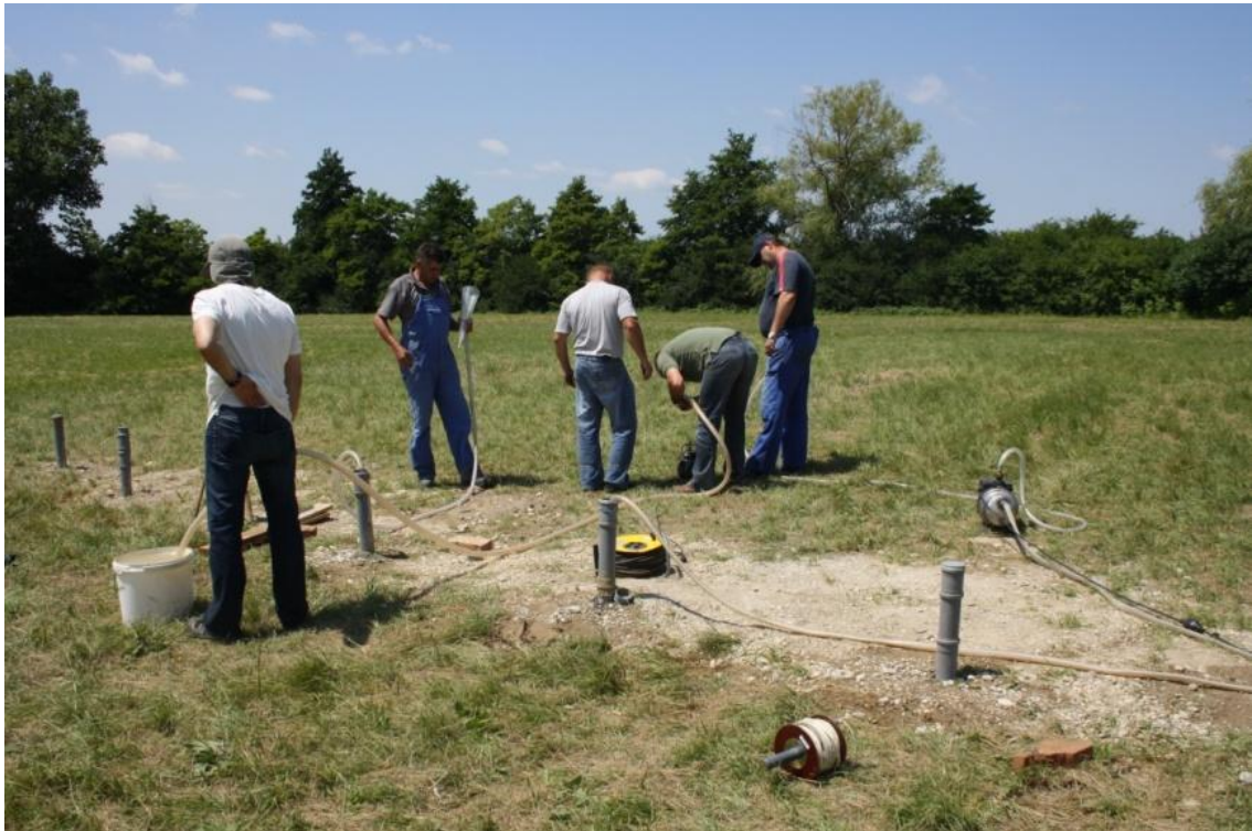
Figure 9 Cleaning of injection and observation wells
