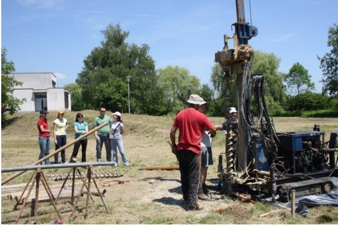
Figure 8 Drilling the boreholes
